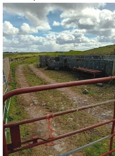
Plate 6. Looking east at existing farm track and cattle crush.
