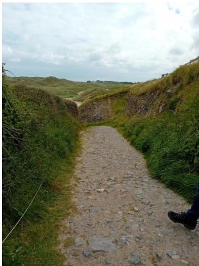
Plate 11. Looking northeast. Top of existing access to be blocked off with stones/embankment and fence.
