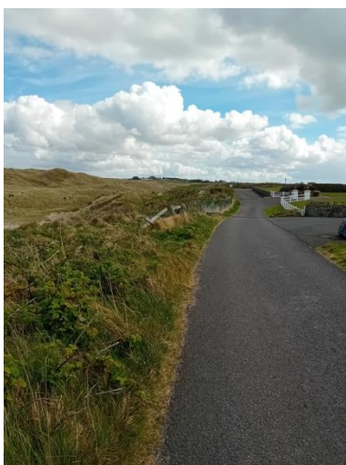
Plate 5. Looking east along existing road: location of new footpath.
